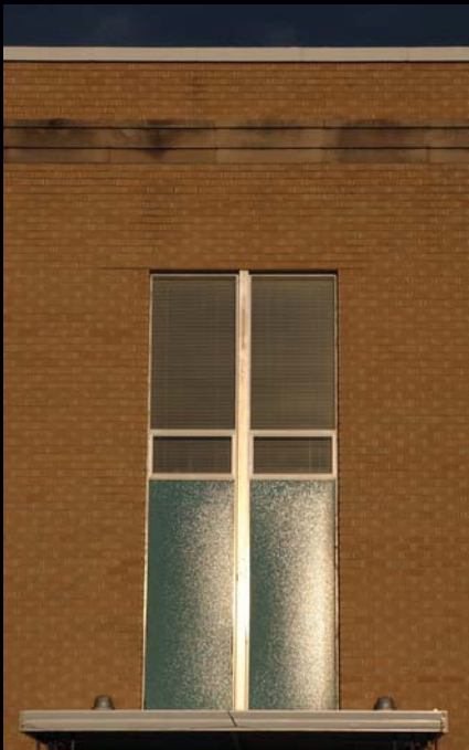
The flat roof of the Upton courthouse is mimicked by the projecting, thin-slab awning over each entryway.
