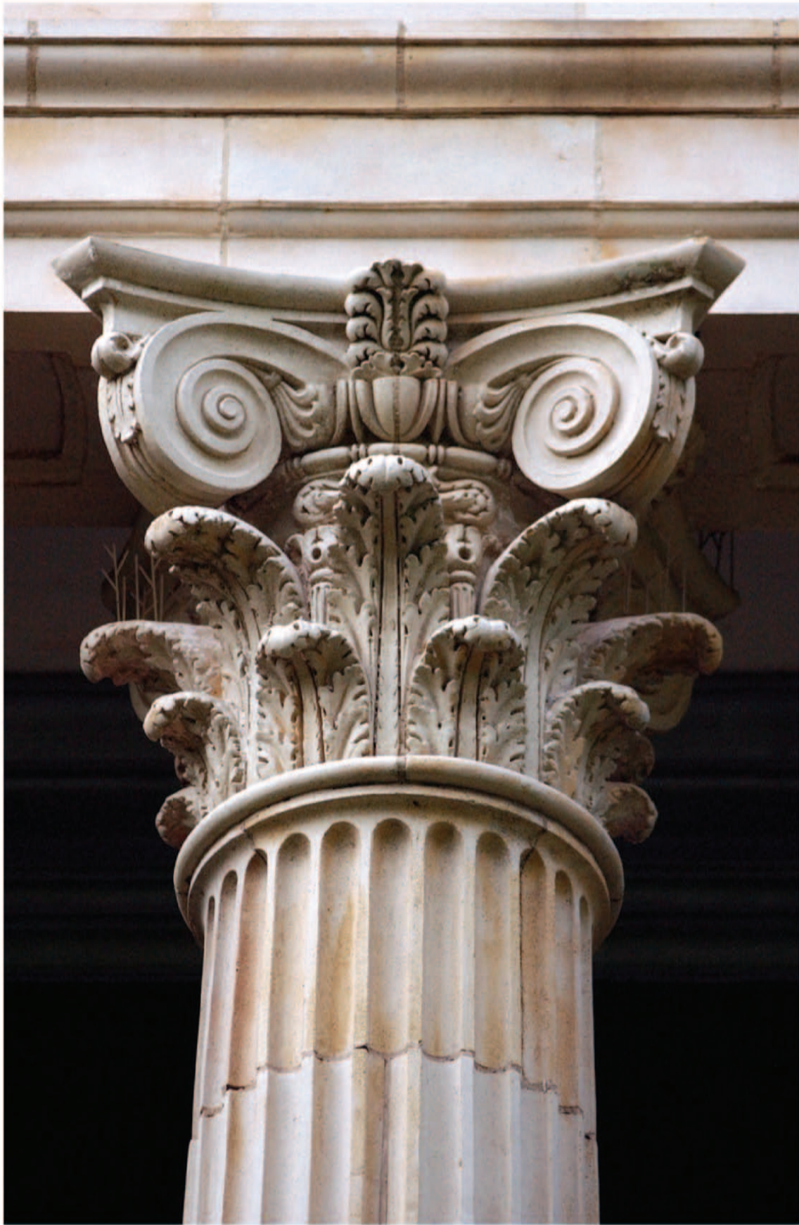
Brooks County boasts one of the best examples of a Corinthian column across all Texas county courthouses. The third and most ornate order of Greek columns (the first two being Doric and Ionic), the Corinthian shaft is slender with shallow vertical grooves, called fluting. The column head, or capital, features volutes (spiral scrolls), and acanthus leaves.
