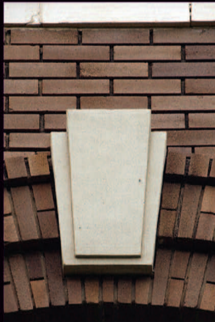
Classical Revival courthouses sometimes incorporate the Roman idea of a keystone above the arched windows.
